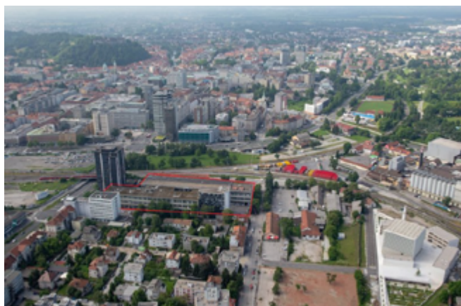
FIGURE: COMMERCIAL, PRODUCTION, AND WAREHOUSE SPACE LIKOZARJEVA IN LJUBLJANA
